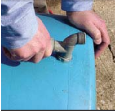
Installing bottom drain
