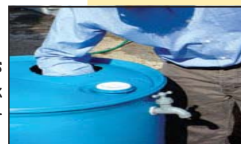
Installing upper drain
